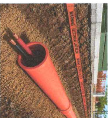
3" PVC PIPE UNDERGROUND CABLE
